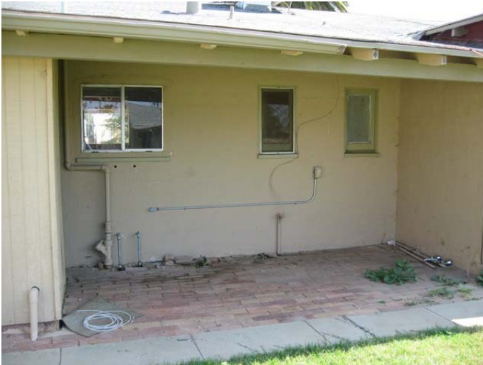
Rear elevation – main house
