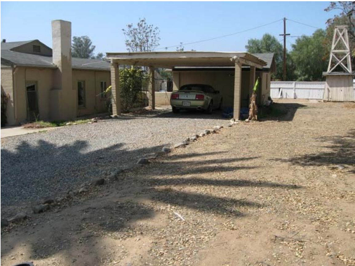
East; Finished garage behind covered parking. New pillars will be installed for the parking structure.
